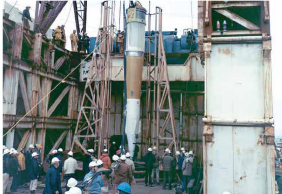
*A Spartan missile body with the nuclear device is lowered downhole for the Cannikin event. The test was successfully conducted on November 6, 1971, on Amchitka Island, Alaska.*
